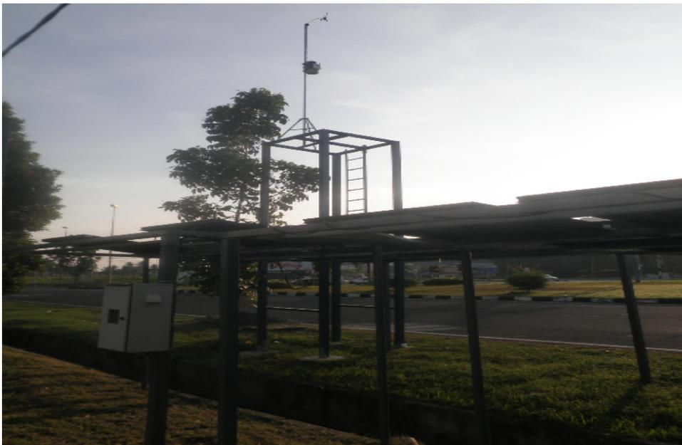
Figure 1: PV array and CERE weather station
