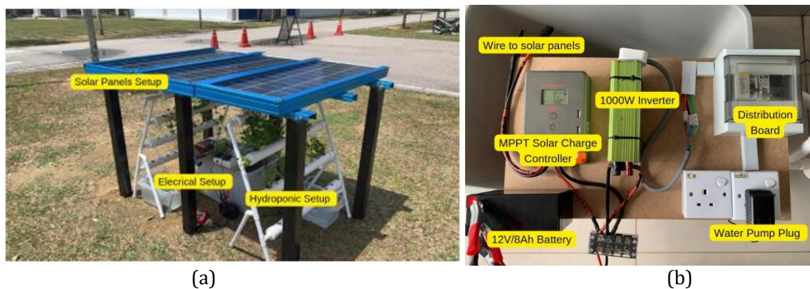
Figure 2. Actual (a) prototype and (b) electrical setup of the system
